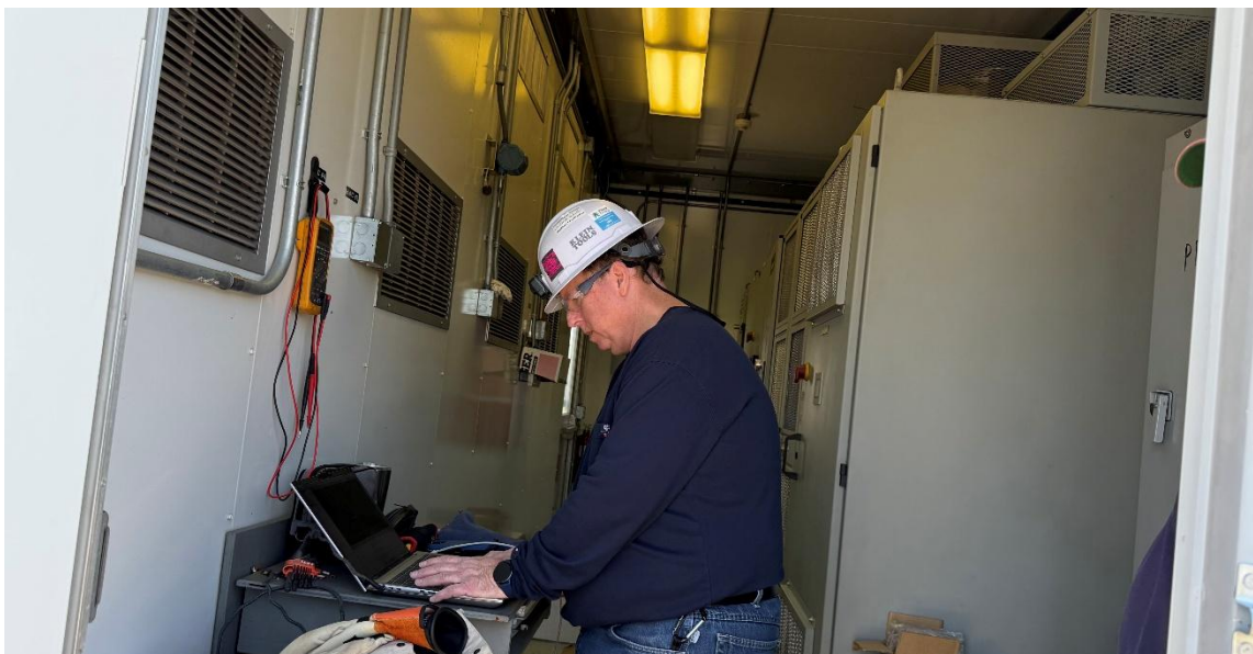
Installation and reprogramming of reconditioned power supply at Sanitary Pump 2
