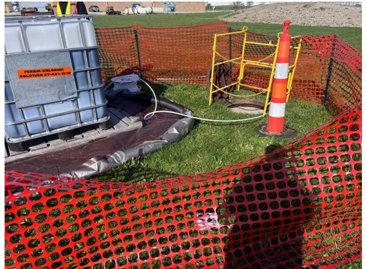
Ferric chloride dosing through PCI-5-MH-101
