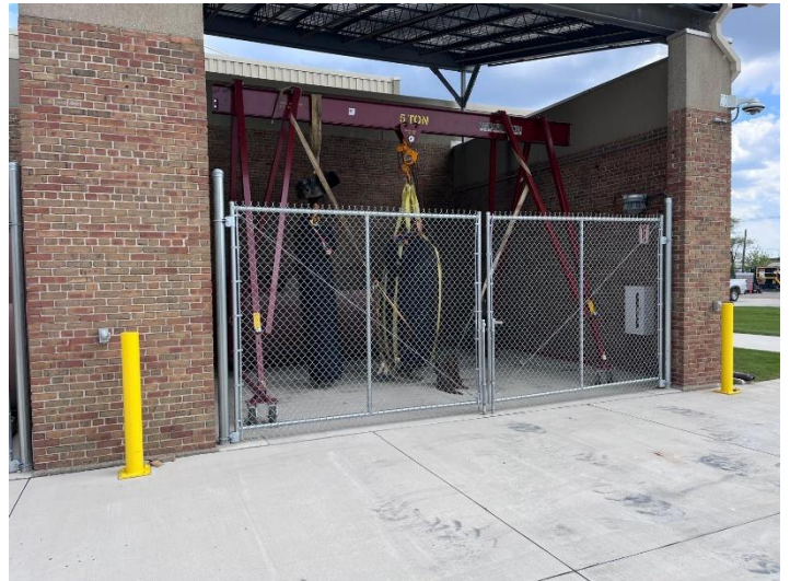
Staging of inflatable plugs for Pumps #3 and 4
