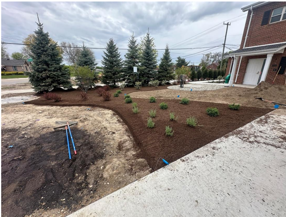
ST-S-1 site landscaping and restoration
