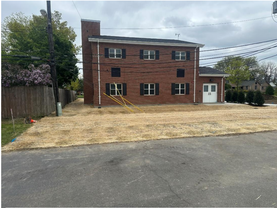
ST-S-1 site landscaping and restoration
