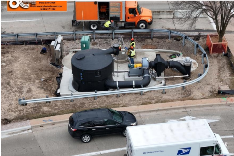
ST-S-1 site status (Aerial view looking north)
