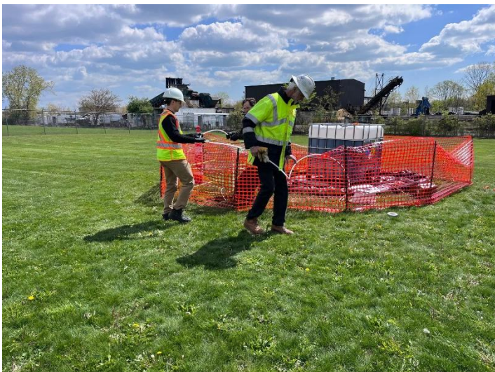
Ferric chloride dosing through PCI-5-MH-101
