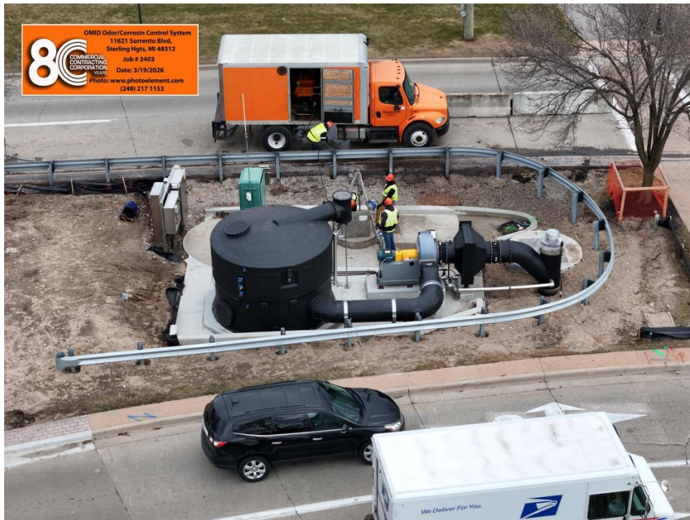
ST-S-1 site status (Aerial view looking north)
