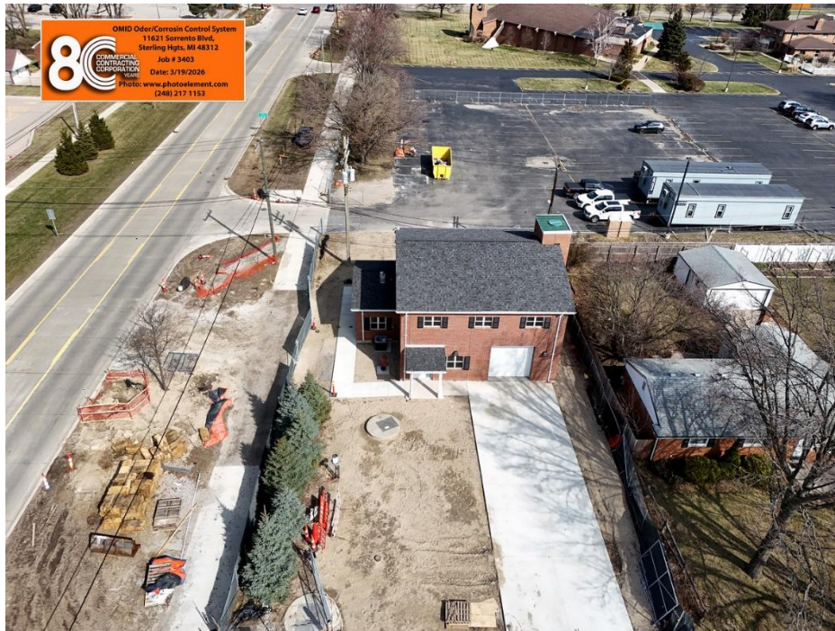
ST-S-3 site status (Aerial view looking at south wall)
