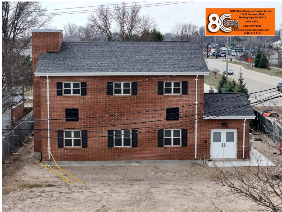
ST-S-1 site status (Aerial view looking at north wall)
