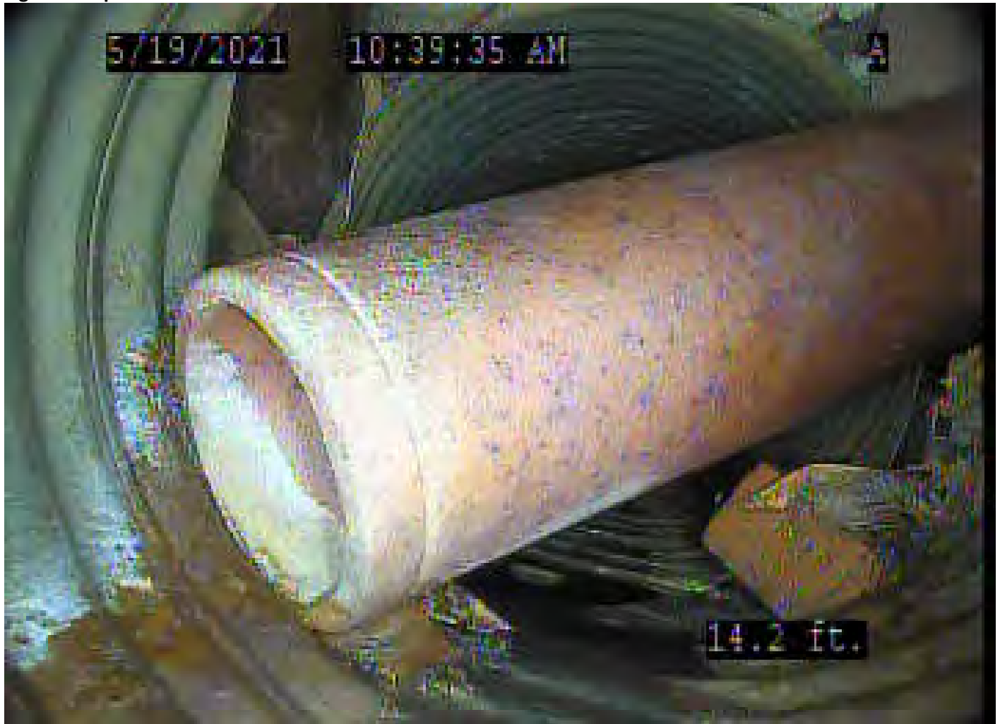
Figure 2. Tap to Storm Drain at 14.2 ft east of BV51-0
