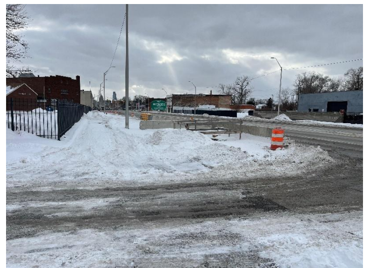
PCI-19-MH-101 jobsite area
