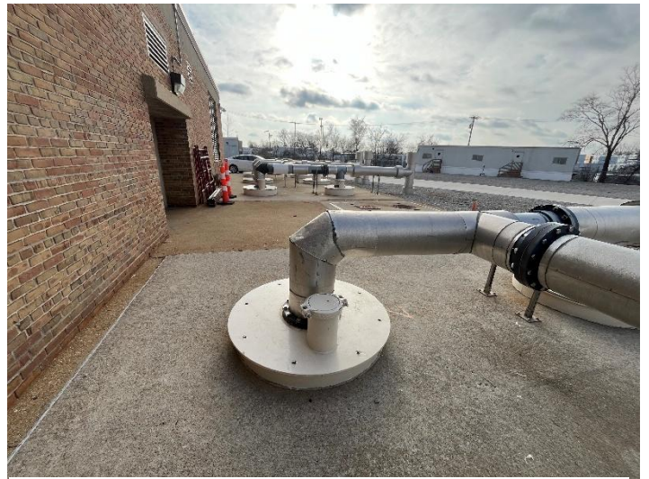
Pump #3 and #4 restored pipe sections
