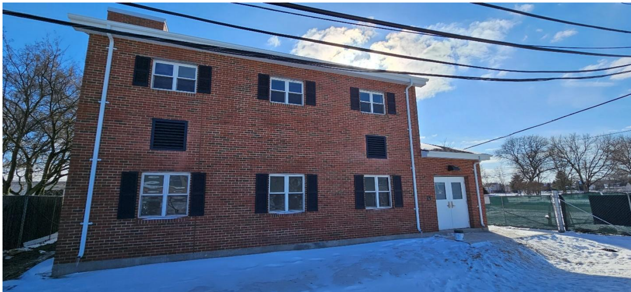
North wall of replica house at ST-S-3 site (looking southwest toward intersection of Dodge Park Road and Sorrento Boulevard)
