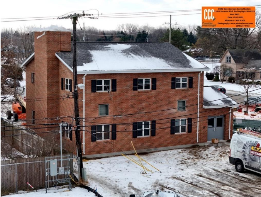
Aerial photo of north wall at ST-S-3 site (looking southwest toward intersection of Dodge Park Road and Sorrento Boulevard)
