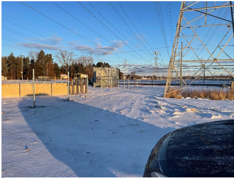
New fence under construction in December, 2025
