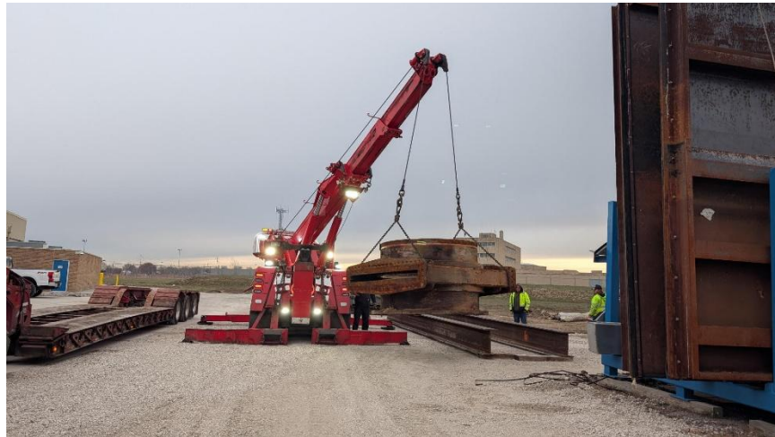
Relocation of stored items to new laydown area
