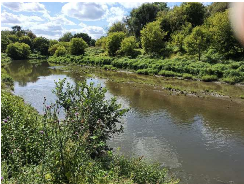
Inspect ID: 2025-10020 Rated Item: 4. Erosion Lat/Long: 42.53224/-83.01526 Caption: 10020 - Unstable slopes and shallow/ shoaled in channel.
