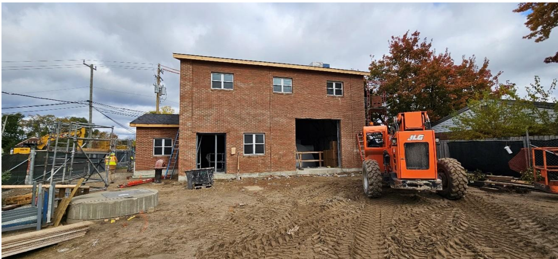
Construction of brick face of south wall at ST-S-3 site (looking north)
