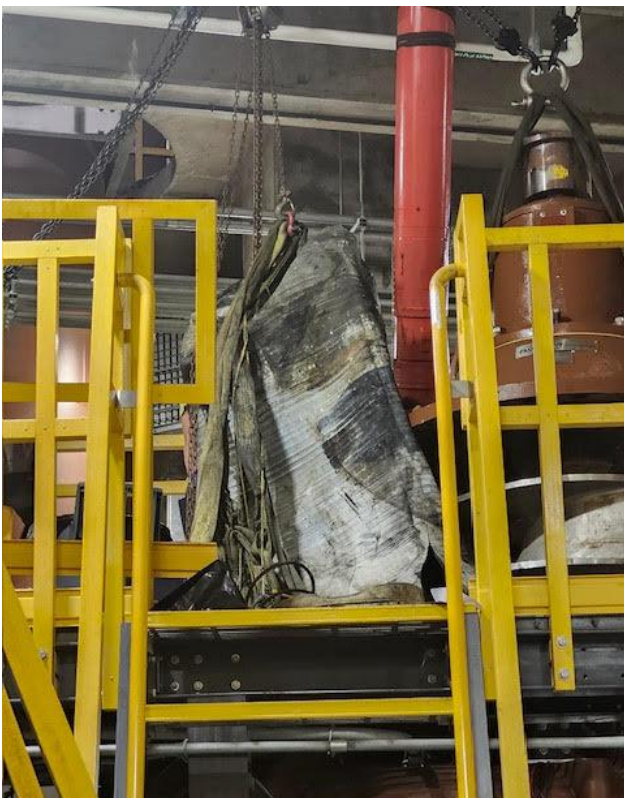
Inflatable plug removed from Pump #3
