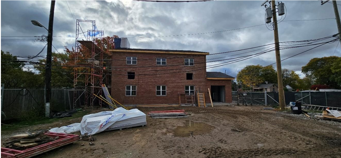
Construction of brick face of north wall at ST-S-3 site (looking south)
