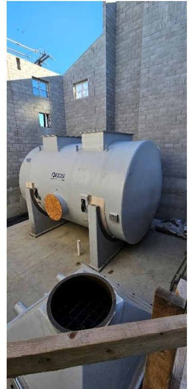
Carbon vessel set on supports in replica house at ST-S-3 (looking northeast)
