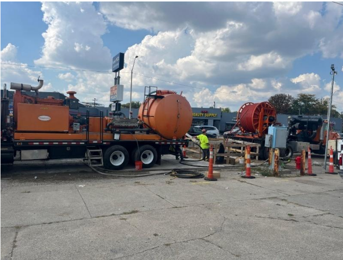
Jet cleaning at PCI-19-MH-102
