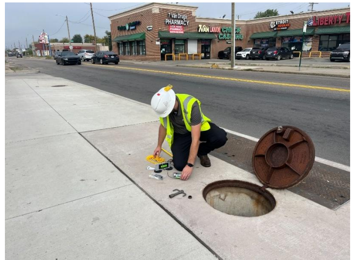
Installation of datalogger at 7 Mile adit structure
