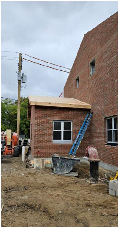
Construction of roof over electrical room at ST-S-3 site (looking north)
