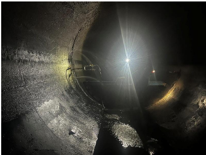
Chemical grouting in PCI-19
