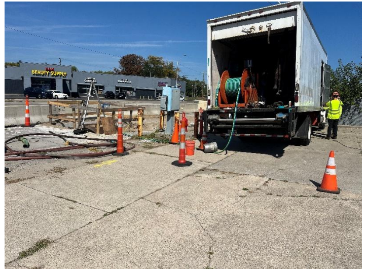
Topside grouting set-up at PCI-19-MH-102
