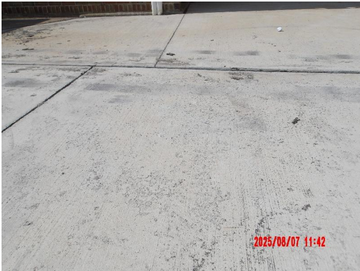
Scaled concrete near wet well mechanical room
