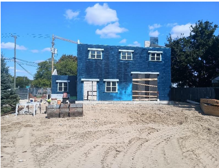
Construction of Replica House CMU walls at ST-S-3 Site (Dodge Park/Sorrento). (L: looking north, R: looking south)
