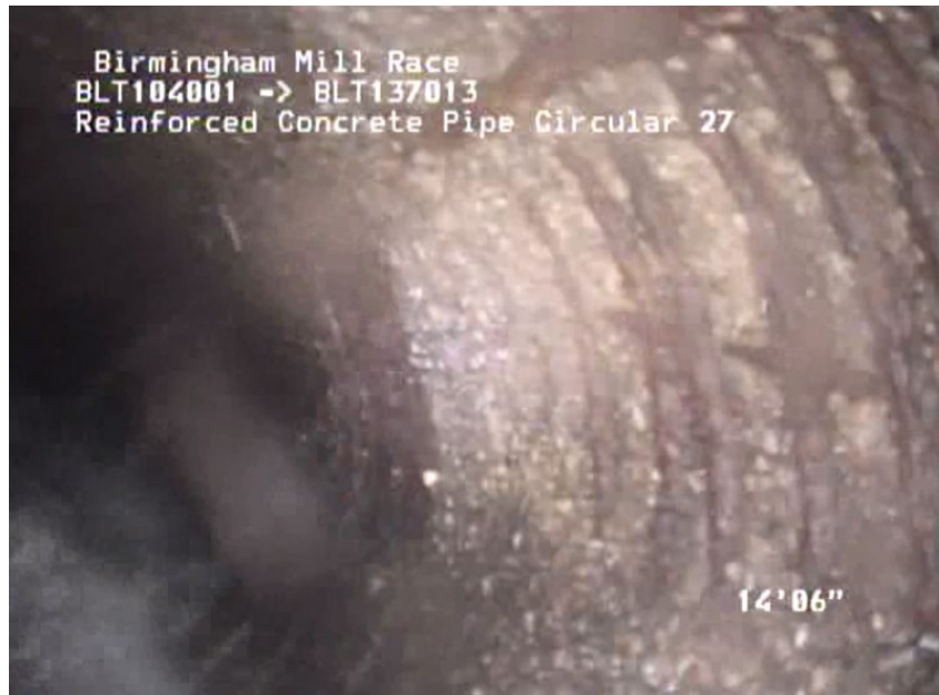
Exposed Reinforcement
