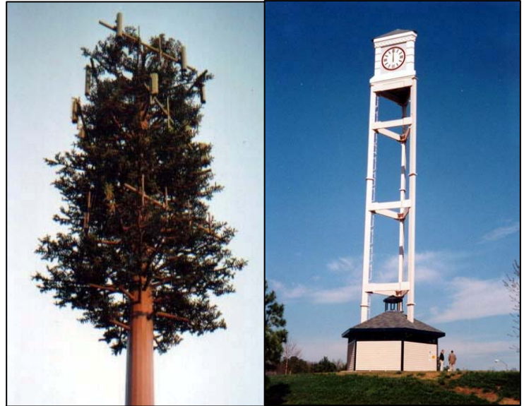
Communication Tower disguised as a tree and clock tower
