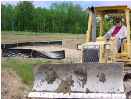
Silt fencing on-site
