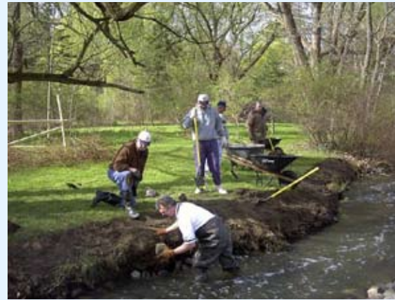
Pebble Creek Stabilization Project
