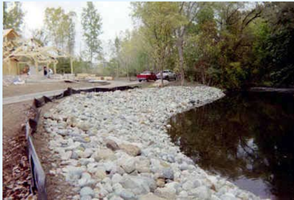
These cobbles were installed as part of a stream bank stabilization effort in a city park in the City of Auburn Hills along the Clinton River.
