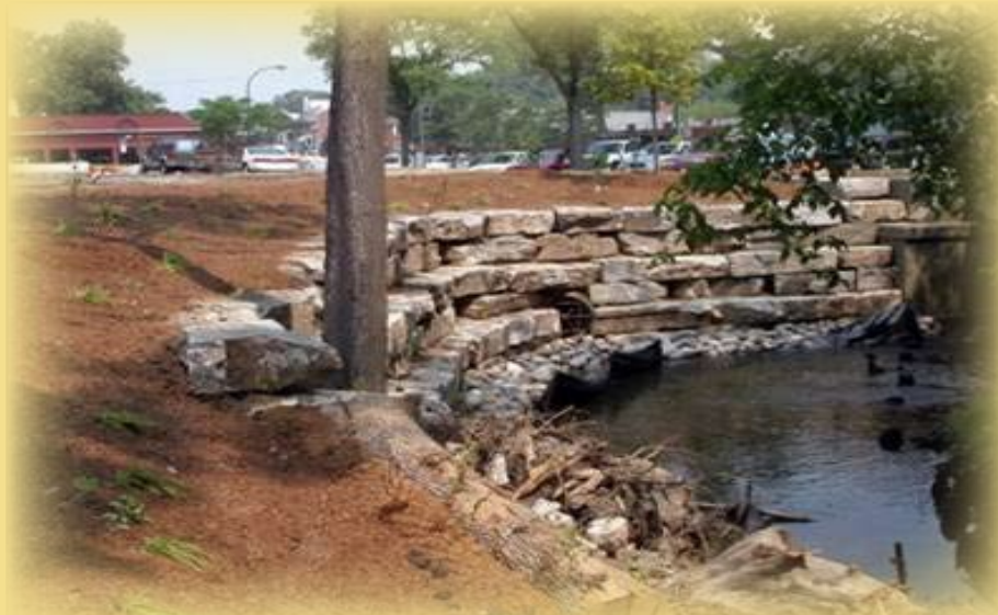
Streambank Stabilization at Quarton Lake Pk
