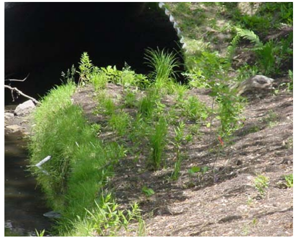
Detail of a portion of the newly planted riparian buffer. Once established, the plants will provide valuable erosion control at the site.
