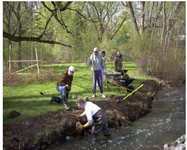
Volunteers install rock to stabilize toe before installing live fascines
