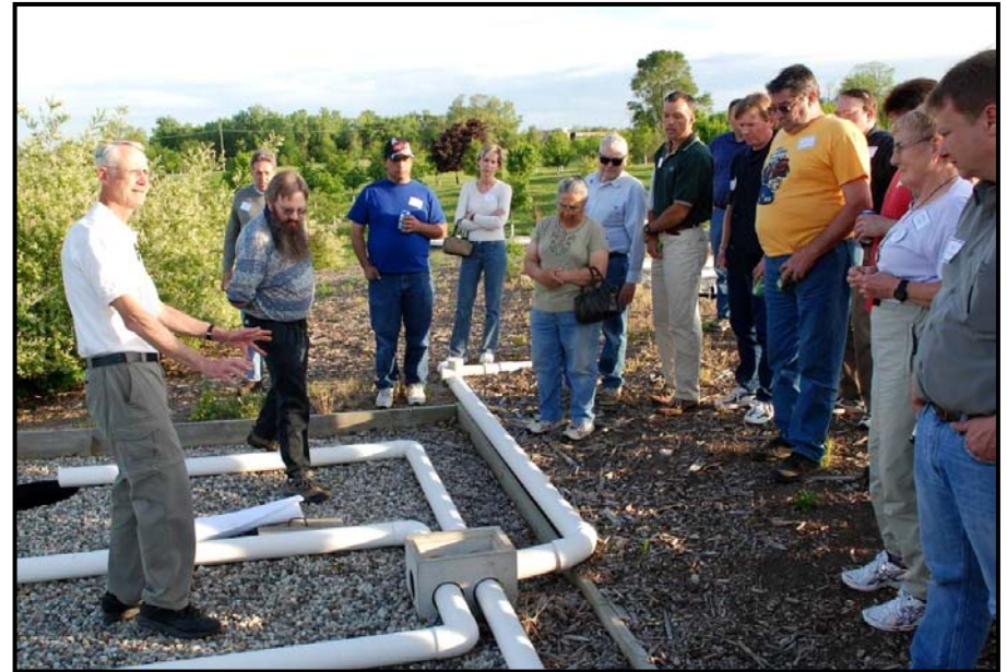
MSU Professor Emeritus Ted Loudon showing participants the underground infrastructure of a septic system.
