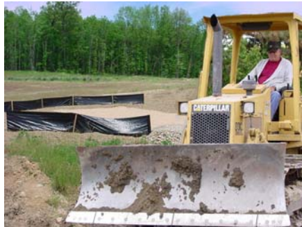
Silt fencing on-site
